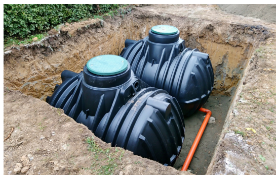
An example of a rainwater harvesting tank
